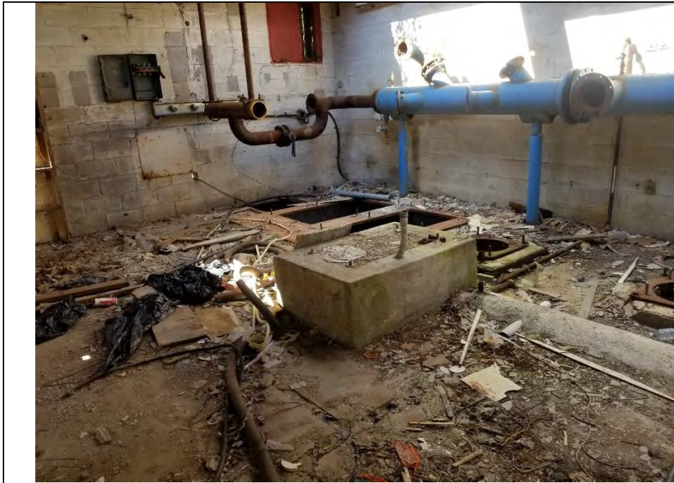
Photo 9: Small concrete block building at 6225 Progress Street, water treatment, contains debris
