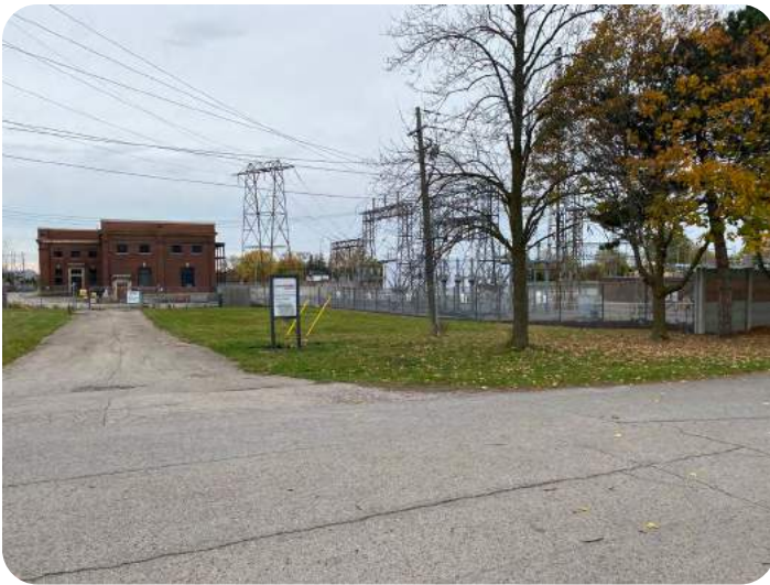
OPG Plant looking south
