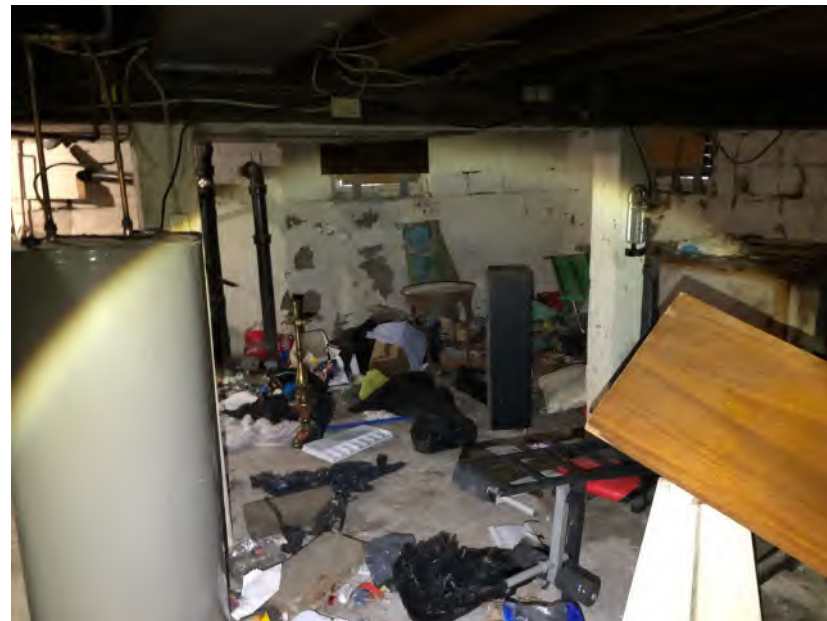
View inside basement of 6285 Main Street facing south
