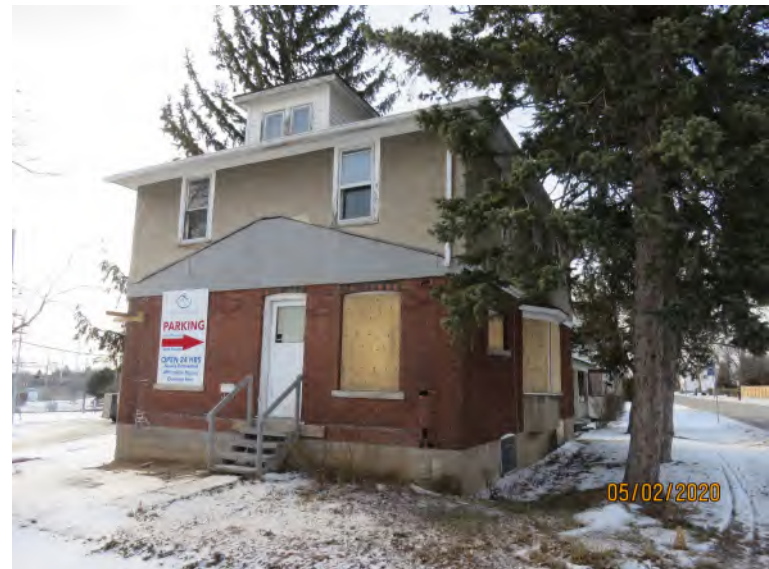
East and north elevation of 5619 Murray Street, facing west
