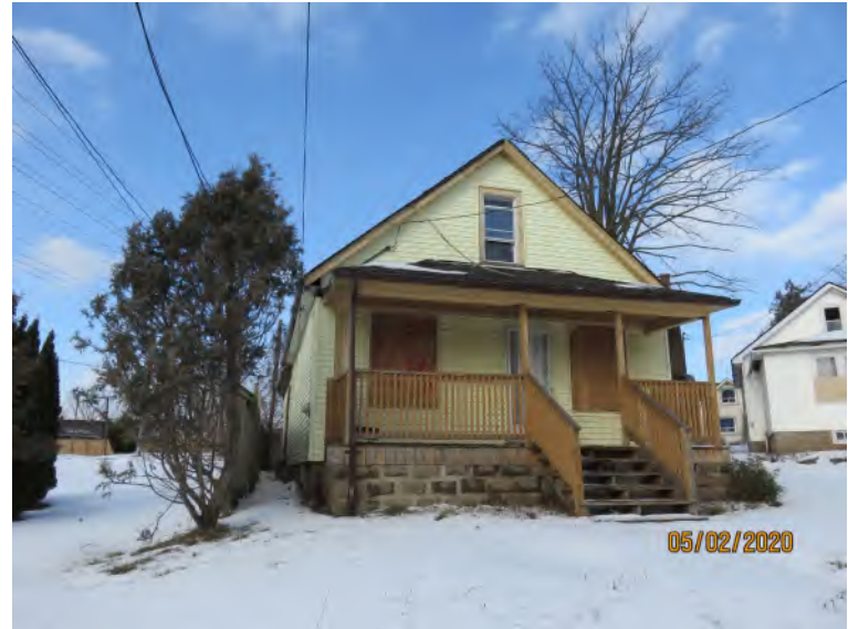
View of dwelling at 5643 Murray Street, facing north
