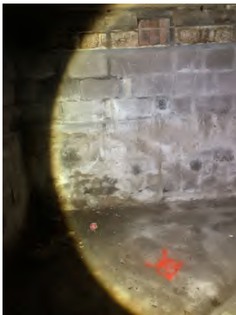
Former tank location inside northwest portion of basement of 6289 Main Street
