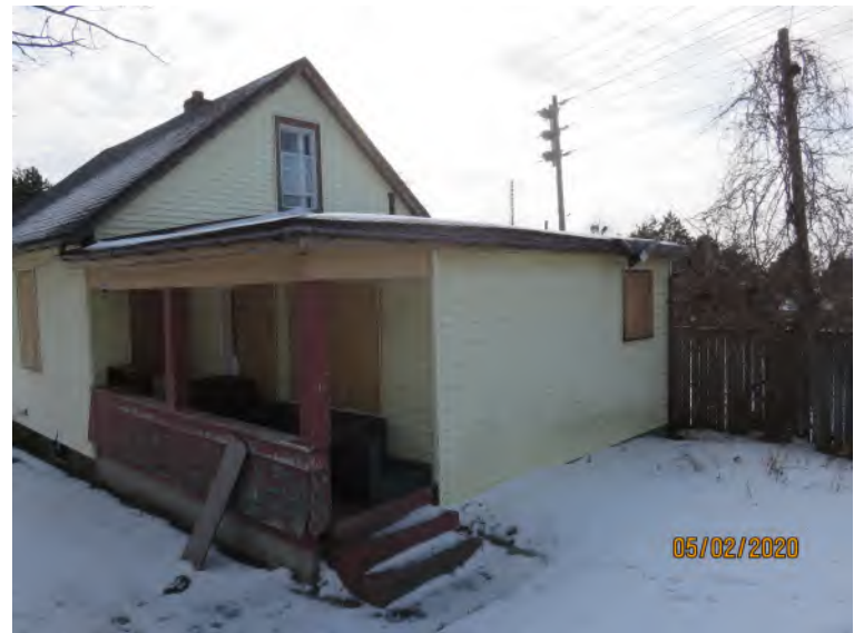
View north elevation of 5643 Murray Street
