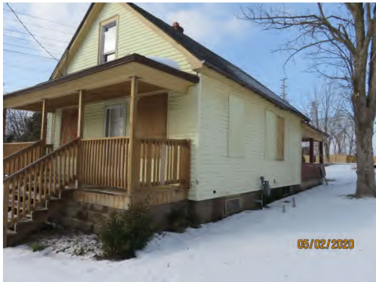
East elevation of 5643 Murray Street facing north
