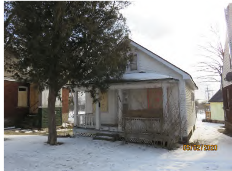
Front elevation of 6289 Main Street, facing south
