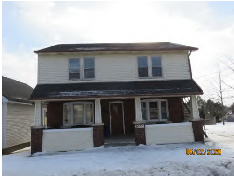
Front elevation of 6285 Main Street, facing south
