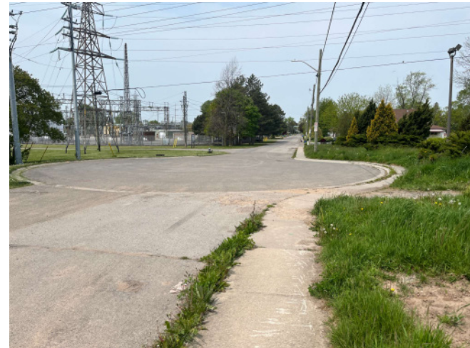
View facing southwest, with hydro station in the background
