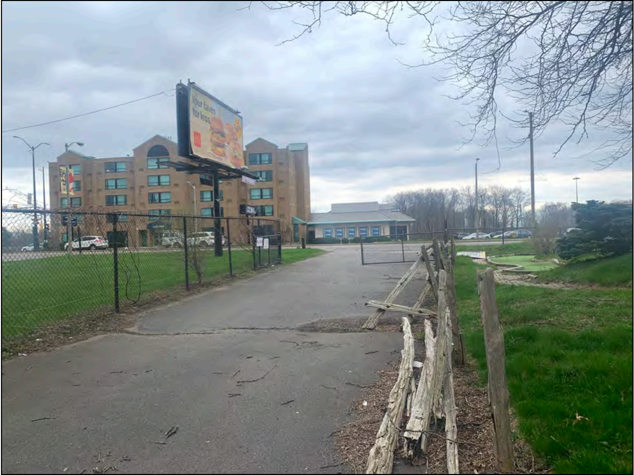
Photograph of the asphalt driveway at the entrance of the site
