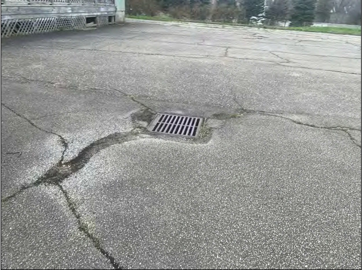
Photograph of a catch basin located on the asphalt surface
