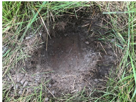
Image 11: Typical test pit found in the northern portion of the subject area showing disturbed soils.
