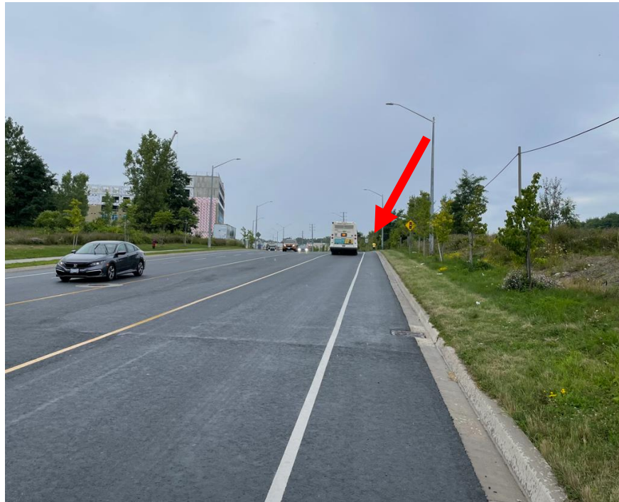
Red arrow indicates location of the proposed south Site Access.
