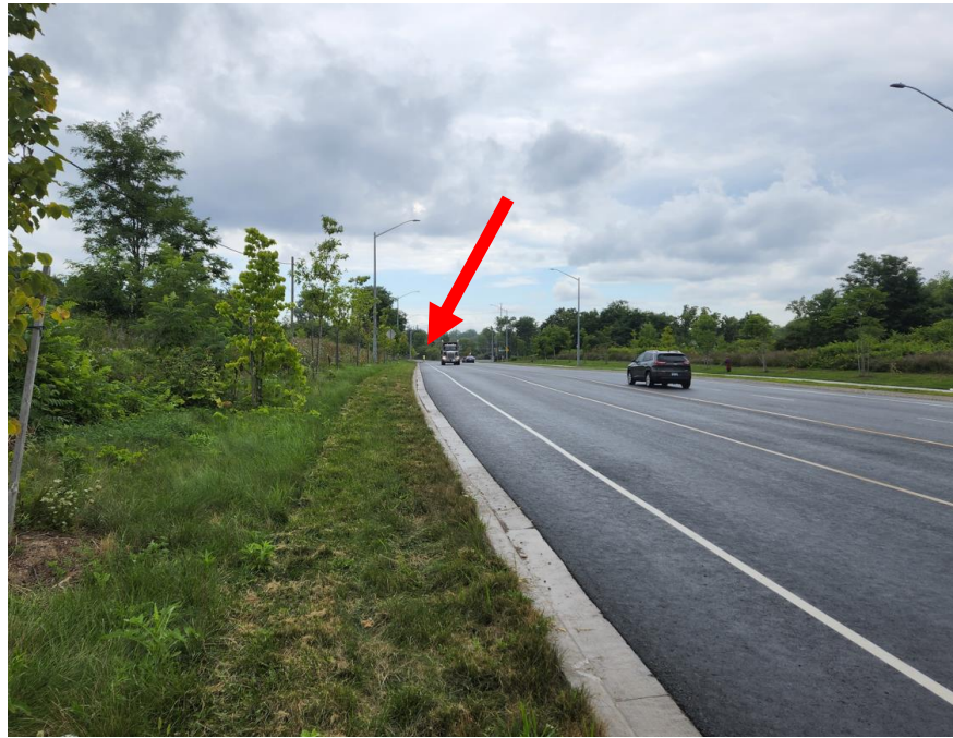
Red arrow indicates the specific intersection sight distance required (160m)
