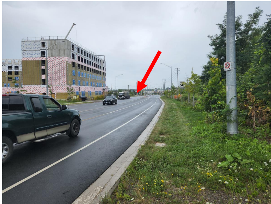
Red arrow indicates the specific intersection sight distance required (160m)
