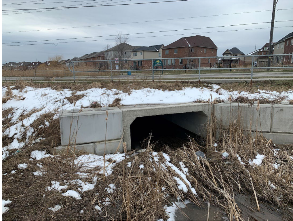
Photo 11 Culvert along western Site boundary, March 2022.
