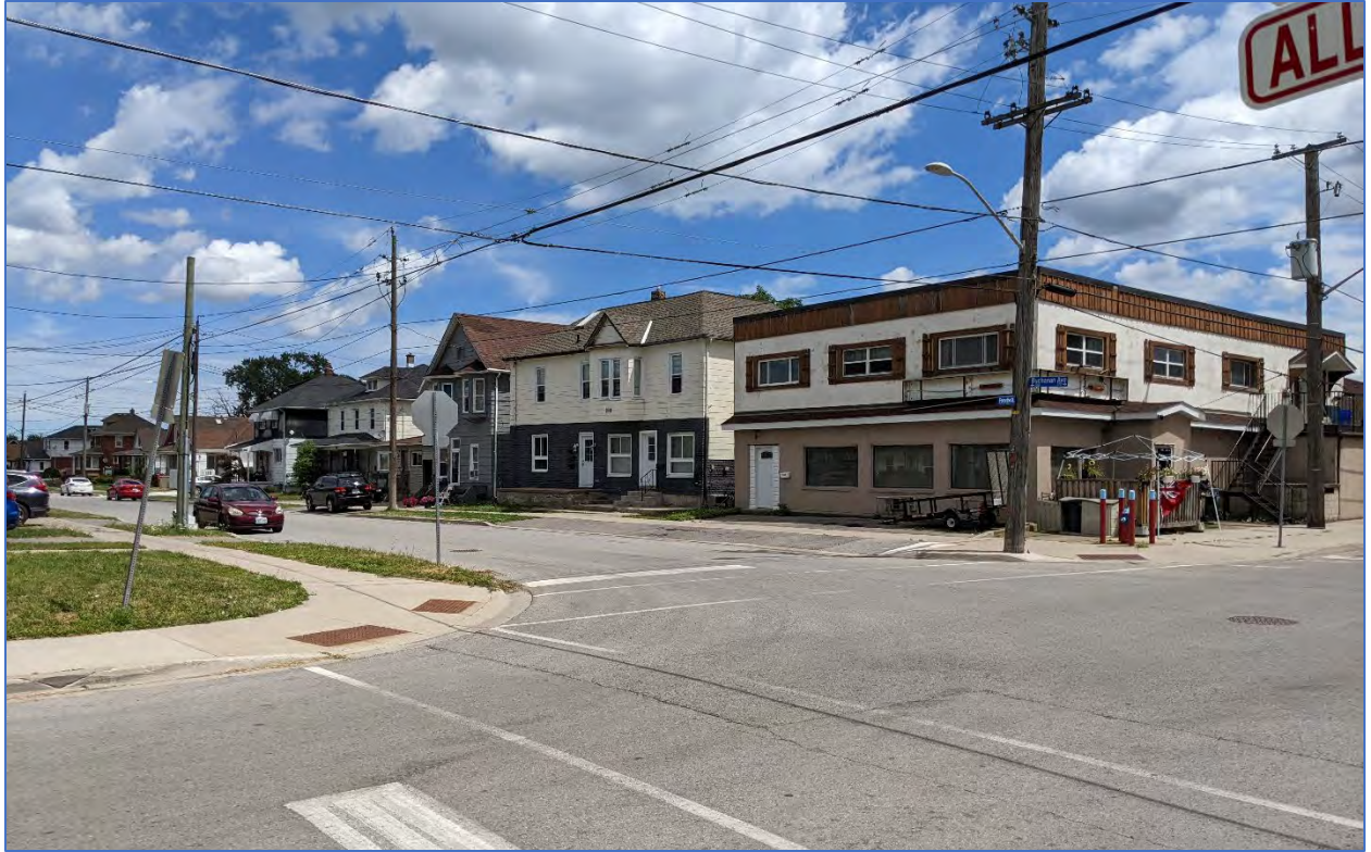
Photo 3: View north at Buchanan Avenue and Forsythe Street intersection.
