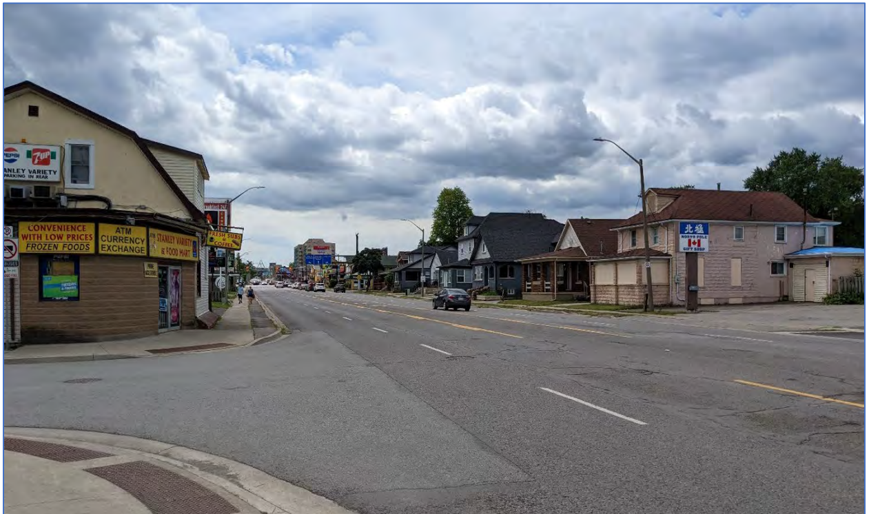
Photo 4: View south on Stanley Avenue towards Ferry Street.
