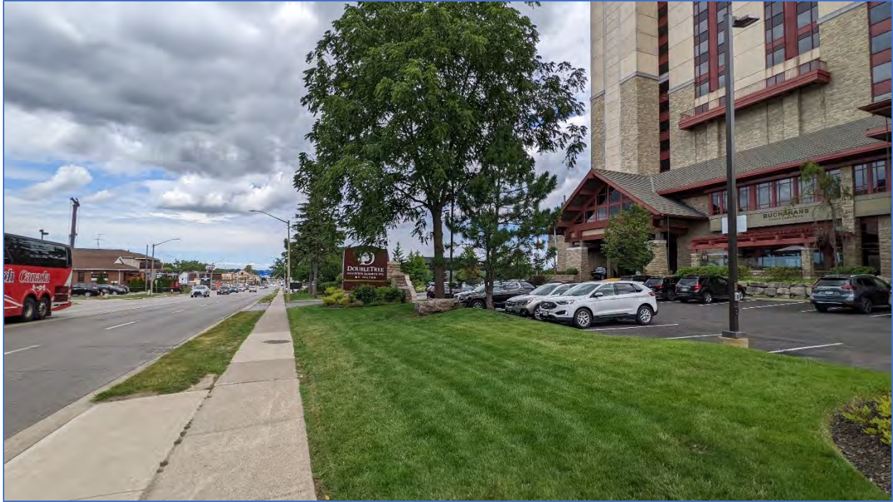
Photo 9: View north towards the Property from 6039 Fallsview Boulevard.
