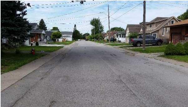
Plate 11: [W] view of Ash St.; proposed sewer is within disturbed ROW, no potential
