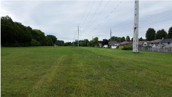
Plate 1: [E] view of hydro corridor; proposed sewer follows existing infrastructure and is disturbed, no potential
