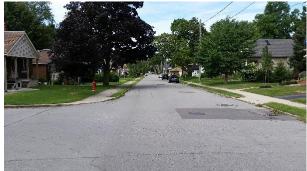
Plate 16: [W] view of Symmes St.; proposed sewer is within disturbed ROW, no potential
