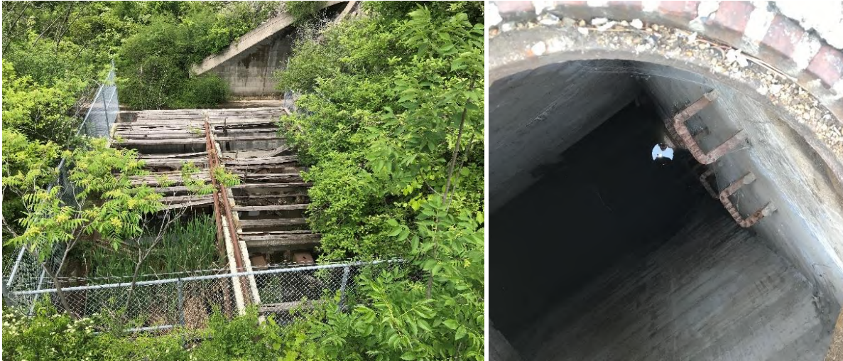
Figure 6.3: McLeod CSO/SSO Tank and Control Structure
