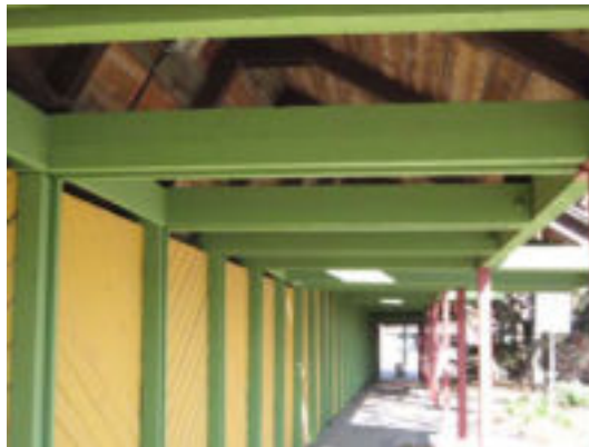
Painted wood shows sign of internal rot
