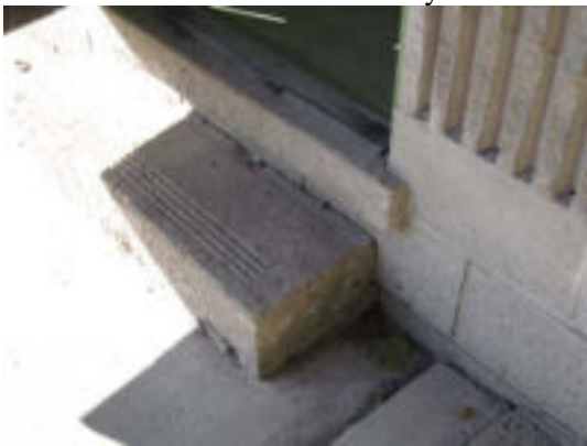
Inaccessible steps into washrooms
