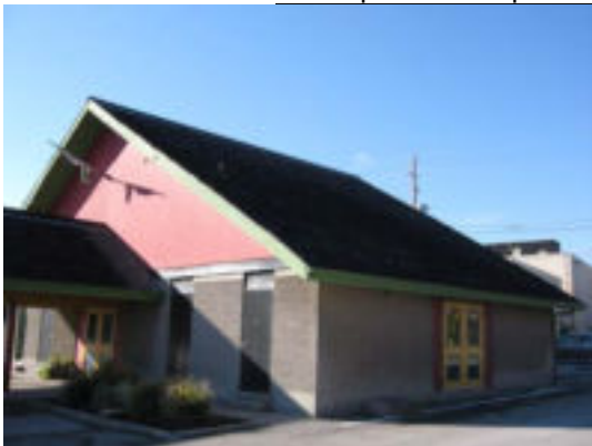
Block wall base; timber roof
