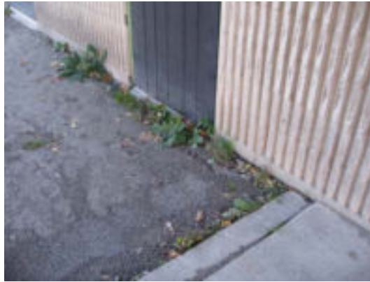
Mud & debris build up at north side of building
