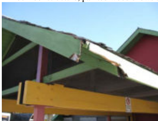
Wood fascia & joists to be repaired/ replaced
