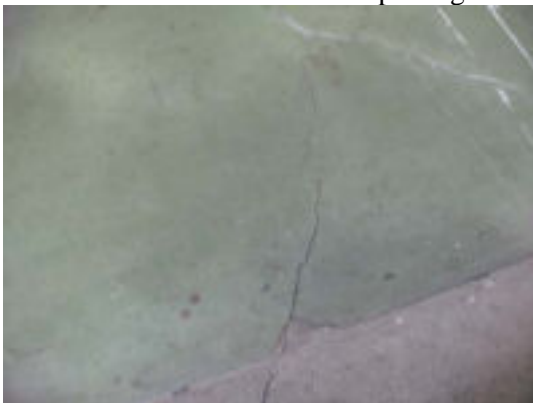
cracks through flooring
