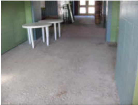
Interior conc. Floor shows signs of spalling
