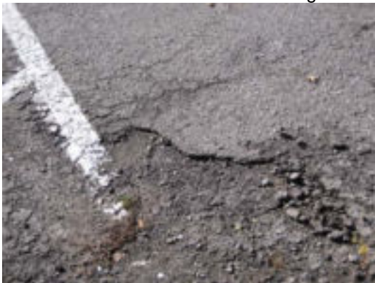
Delaminated asphalt
