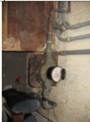
Water meter in Janitor's closet
