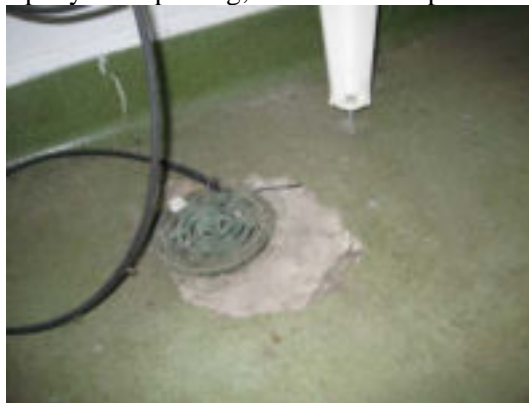
Delaminated epoxy around floor drains
