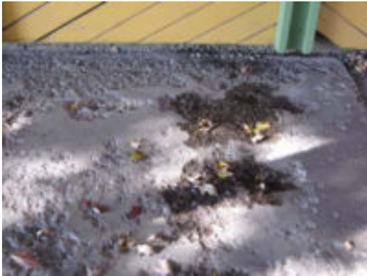
Concrete shows signs of severe spalling
