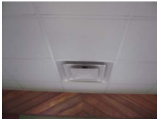
Typical air diffuser
