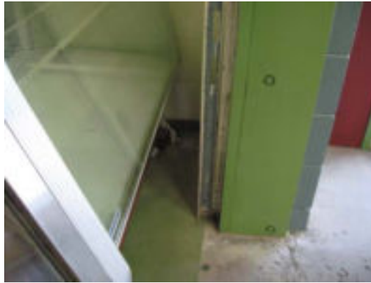
Epoxy floor peeling; concrete floor pitted & cracked
