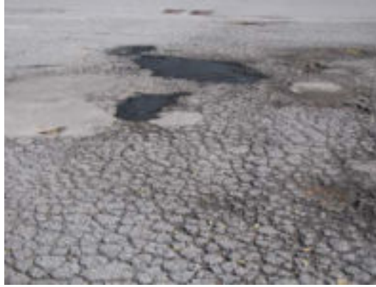
Asphalt surface has potholes & "alligatored" surface
