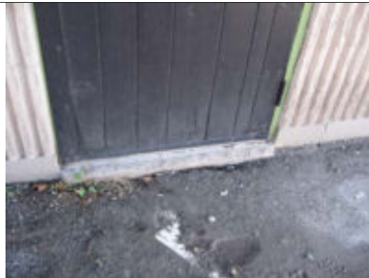
Water penetration & mud build-up at foundation
