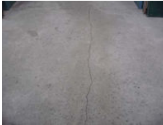
Slab-on-grad concrete floor cracked throughout
