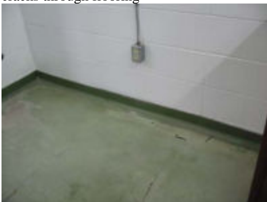
Cracking in tenant floors throughout
