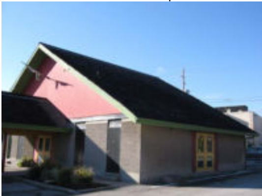
Block wall base & timber structure roof
