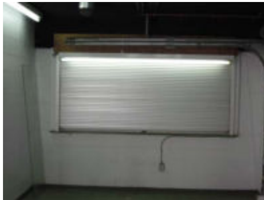
Block walls & rolling o/h doors
