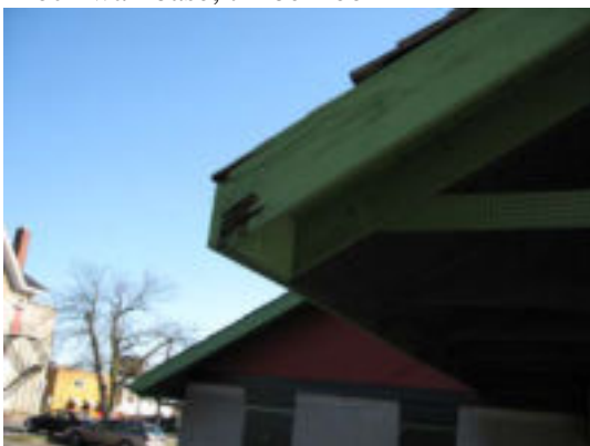
Exterior wood painted w/ sign of rot
