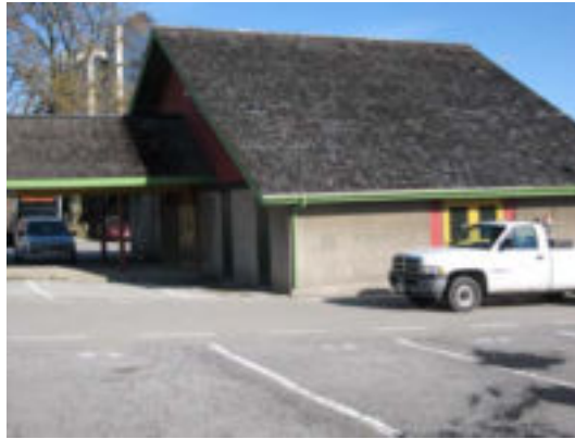
Cedar shakes at end of useful life cycle
