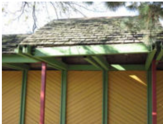
Cedar shakes to be replaced
