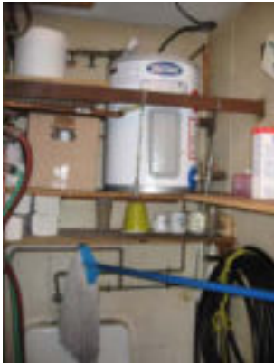
Water heater & slop sink in Janitor's closet / Electrical room
