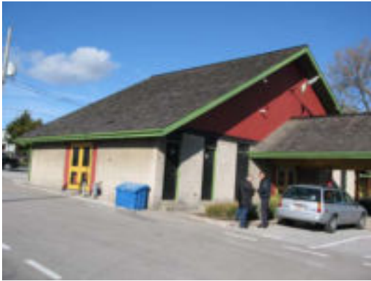
Cedar roof at end of useful life cycle
