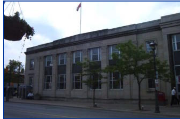
Niagara Falls Post Office Building
