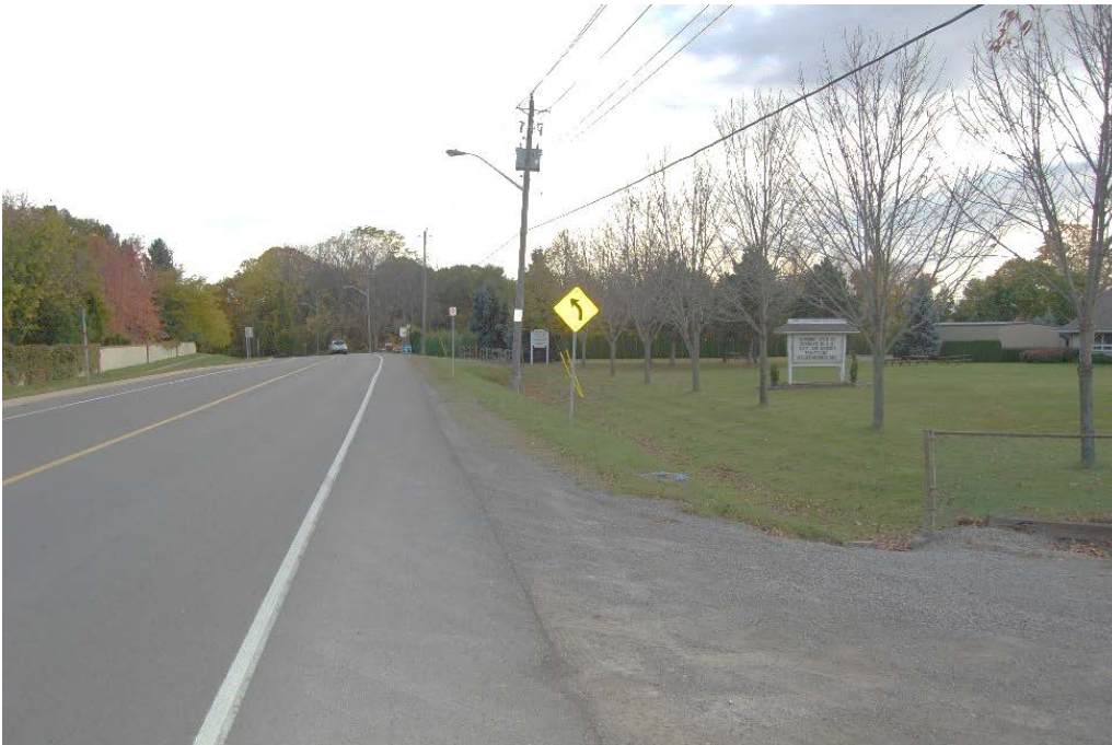
Figure 3: Non-accessible bus stop on a rural road with no landing pad or sidewalk.
