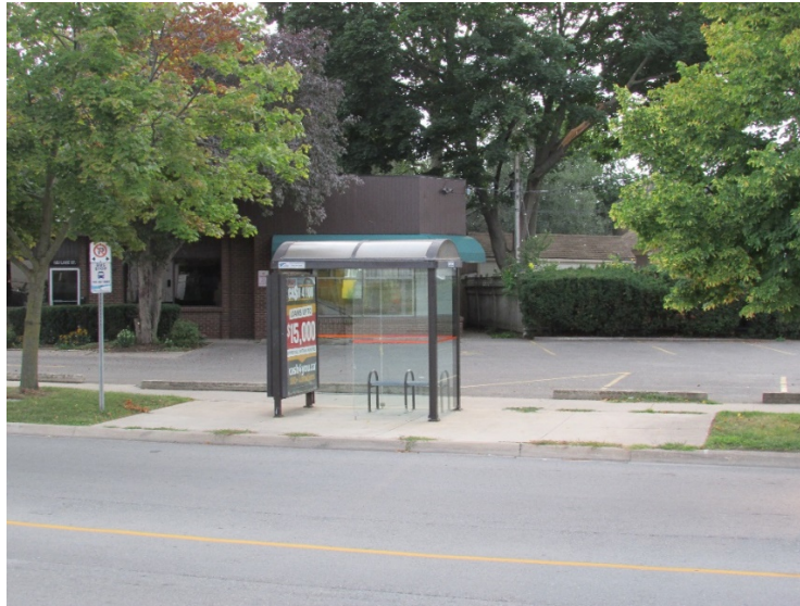
Figure 7: A stop with smooth unobstructed surfaces between the loading area, sidewalk and passenger amenities.
