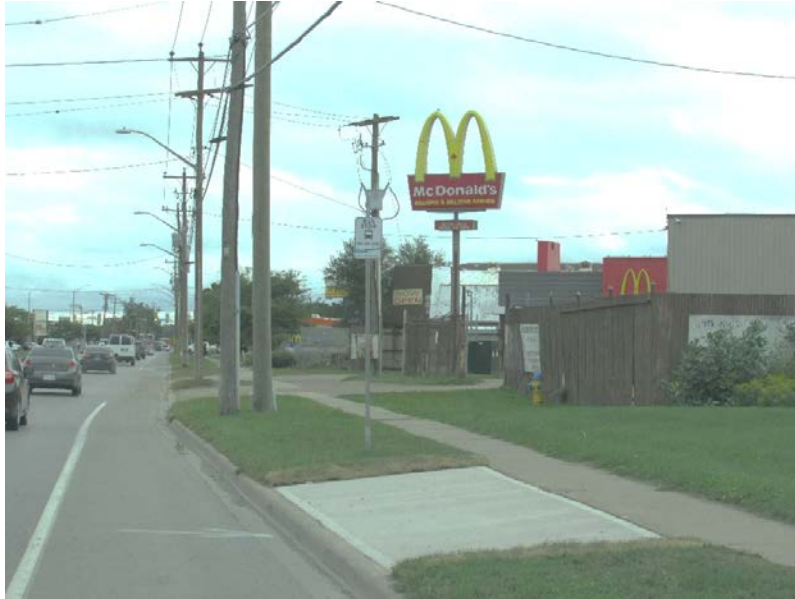
Figure 5: Landing pad is long and deep enough to deploy the ramps and have space to manoeuvre.
