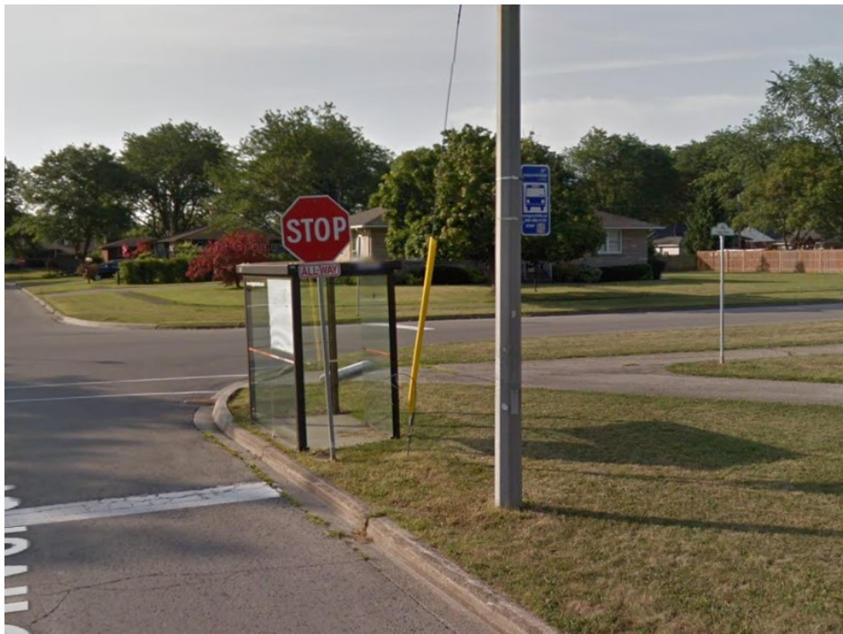
Figure 10: A non-accessible bus stop with a utility guide wire obstructing the landing area with reflective sheath.
