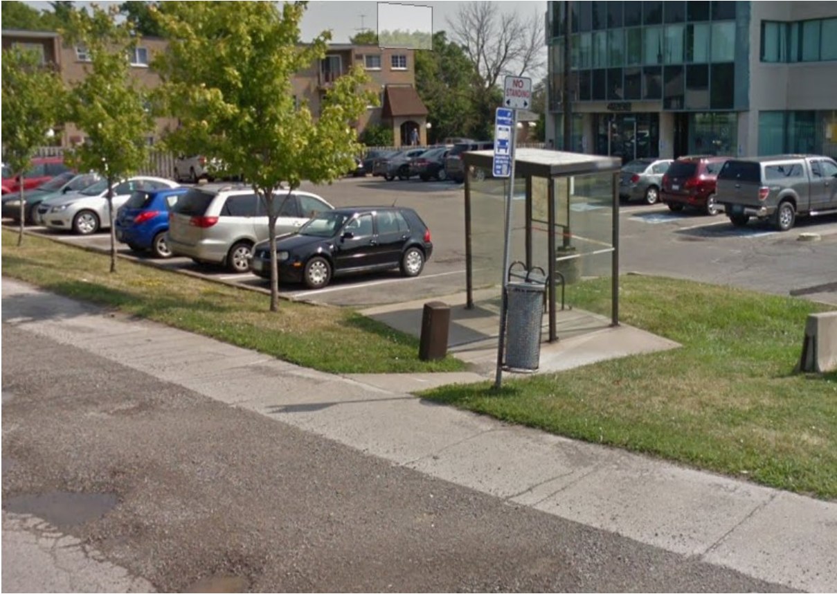
Figure 9: A non-accessible stop with shelter connected to the loading area by a concrete sloped pathway.
