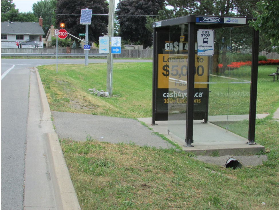
Figure 8: A non-accessible stop which lacks a physical barrier between the deployment area and a steep slope.
