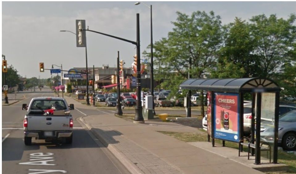
Figure 1: Bus stop on a road with an urban cross section, including municipal sidewalks.
