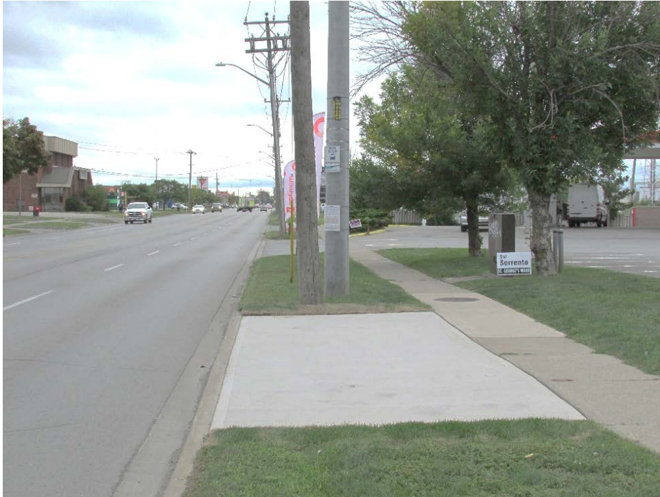
Figure 2: Bus stop on an urban road with a landing pad connected to the sidewalk.
