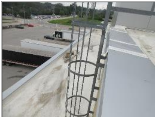
Partial view of the lower roof system.
