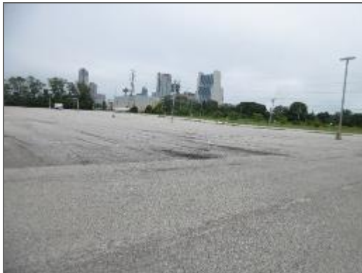
General view of asphalt-paved parking area at the southwest portion of the Site.
