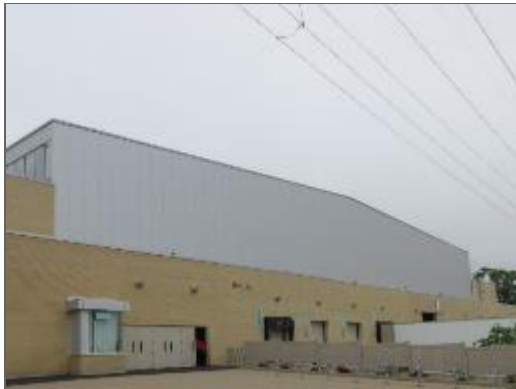
View of the metal wall panels noted on the west elevation of Site Building.
