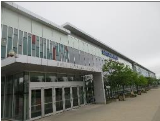
Typical view of the curtain wall systems noted on the north elevation of Site Building.
