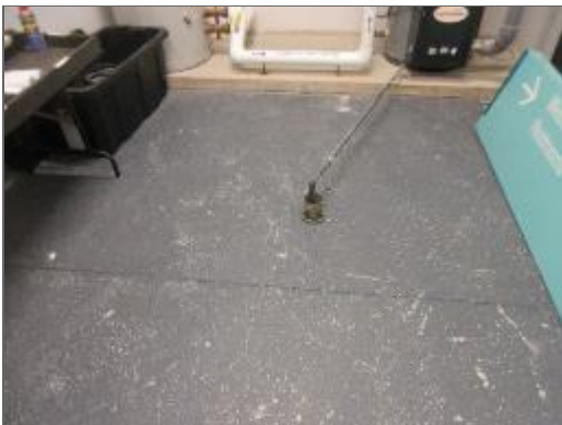
View of typical epoxy coated concrete noted within a mechanical room.
