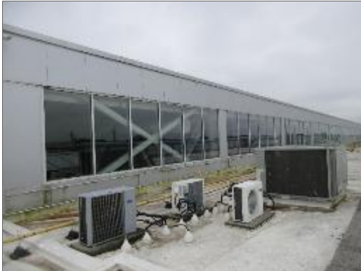
View of the strip window configuration noted on the north elevation of Site Building atop the main roof system.
