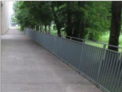
View of typical metal guardrails noted adjacent to the south elevation of the Site Building.
