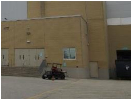
View of a typical punched window noted on the west elevation of Site Building.
