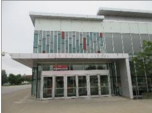
General view of the canopy located on the north elevation of the Site Building.
