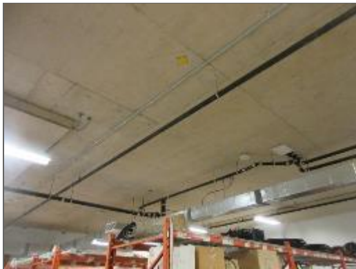
View of exposed concrete within service rooms.
