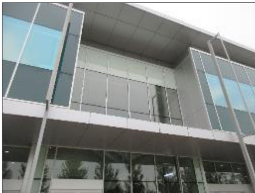
General view of the canopy located on the north elevation of the Site Building.
