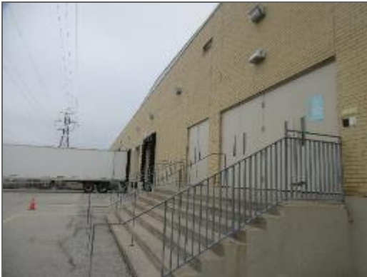
General view of the metal entrance doors on the west elevation of the Site Building.
