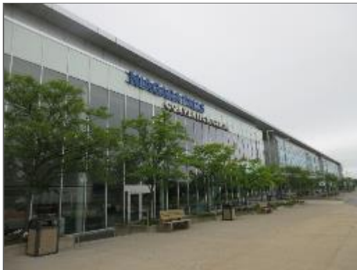
Typical view of landscaping adjacent to the north elevation.
