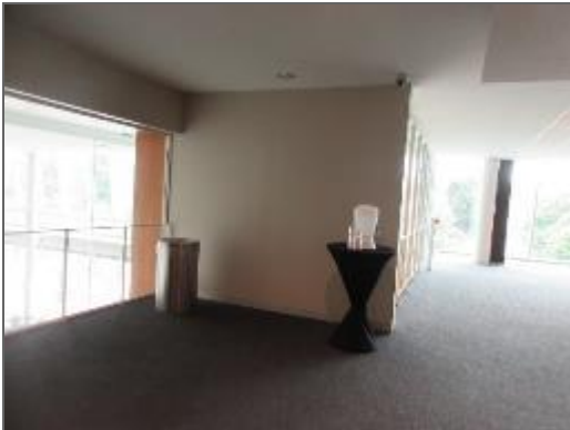
View of the typical wall finishes within the corridors of the Site Building.
