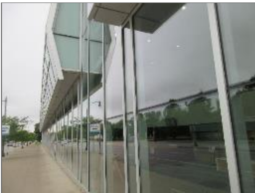
Typical view of the curtain wall systems noted on the east elevation of Site Building.
