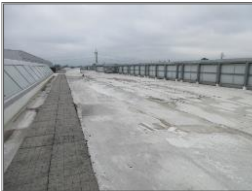
Partial view of the main roof system.
