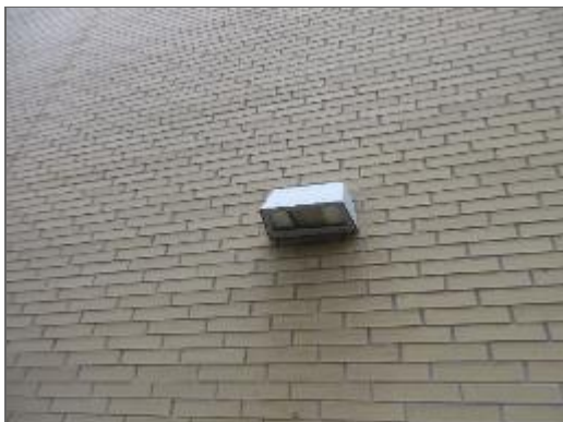
Typical view of exterior lighting at the Site Building.
