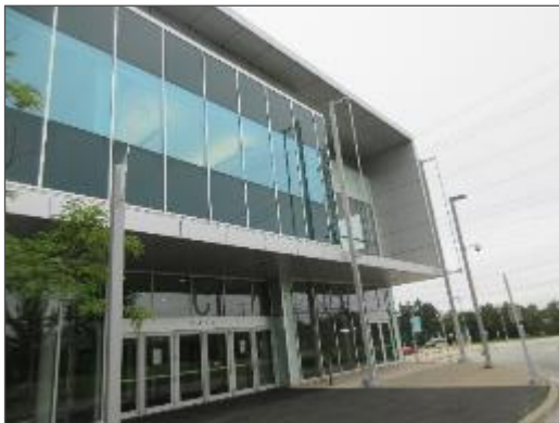
General view of the canopy located on the north elevation of the Site Building.
