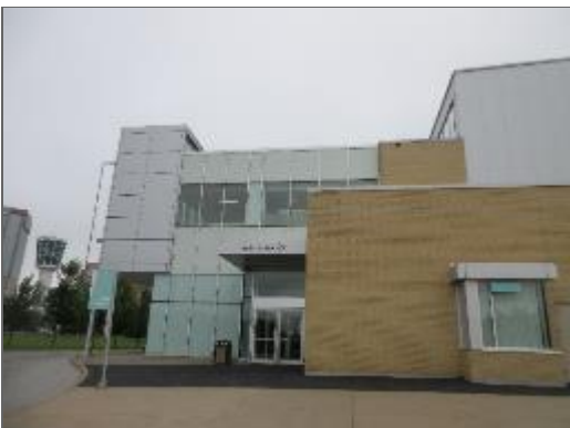
General view of the canopy located on the west elevation of the Site Building.
