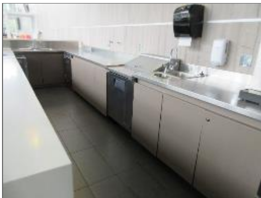
Typical view of millwork within a café.
