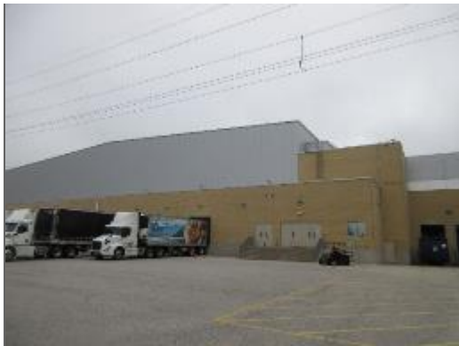
View of the brick veneer masonry on the west elevation of Site Building.
