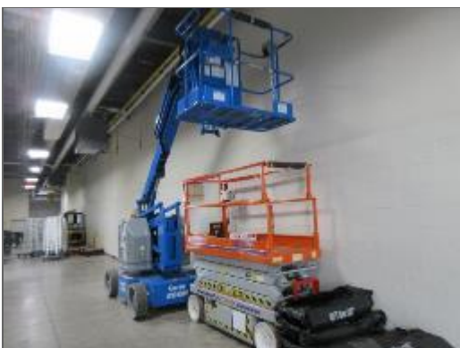
View of the typical painted concrete block within a service area.
