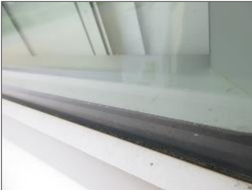
View of window glazing seals.
