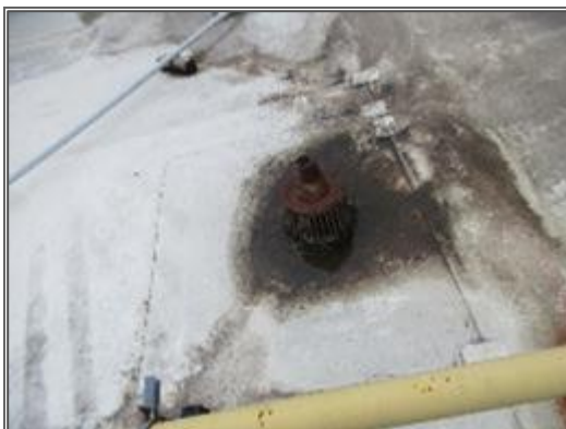
Typical view of a roof drain.
