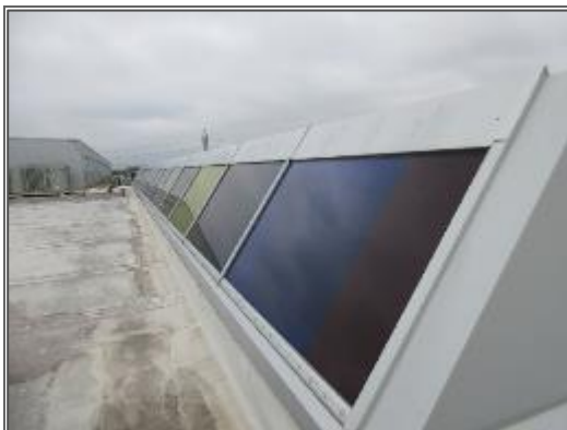
General view of a typical sloped skylight on the roof.
