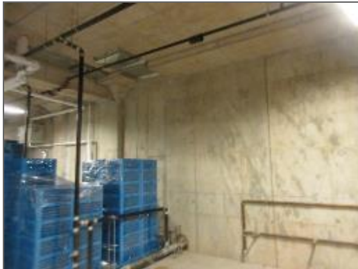
View of typical wall finishes within the basement of the building.
