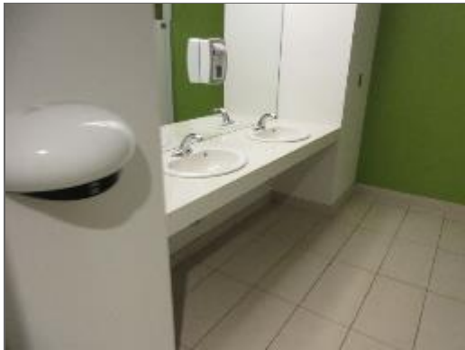
View of millwork within a washroom.
