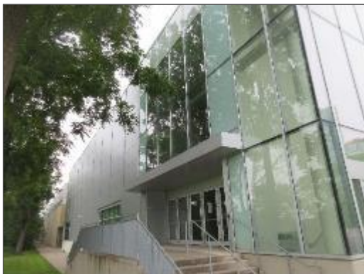
General view of the canopy located on the south elevation of the Site Building.
