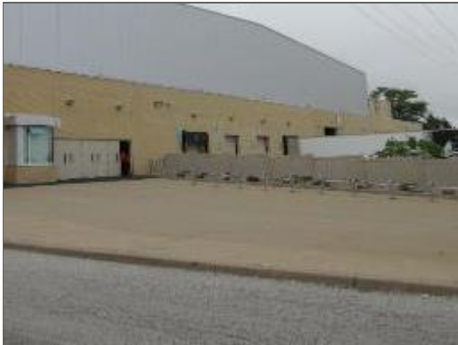
View of the concrete walkway adjacent to the west elevation of the Site Building.
