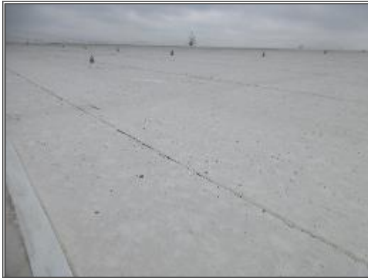
Partial view of the upper roof system.
