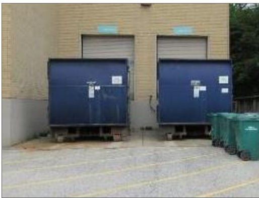
View of the concrete pad at the garbage area adjacent to the west elevation of the building.
