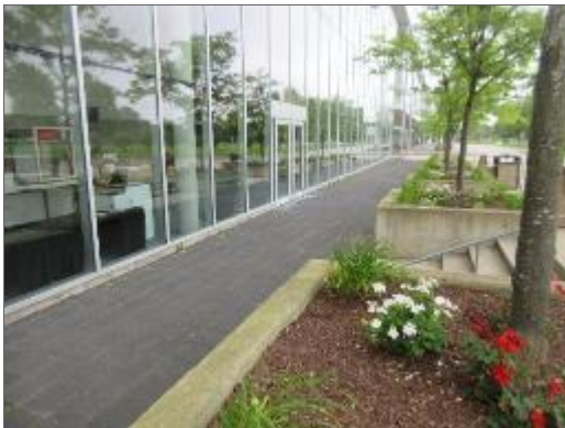
View of the concrete paver walkway adjacent to the north elevation of the Site Building.
