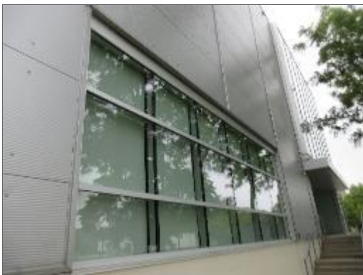
View of a typical punched window noted on the south elevation of Site Building.
