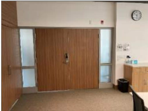
View of typical interior doors within the building.
