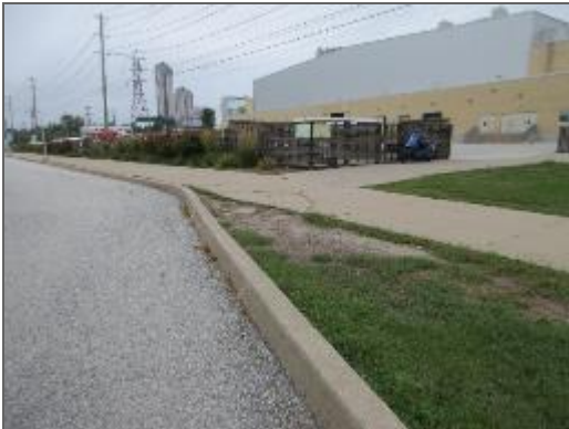
Typical view of concrete curbs within the Site.
