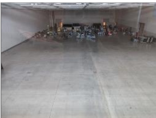
View of exposed concrete flooring noted within an exhibition hall.
