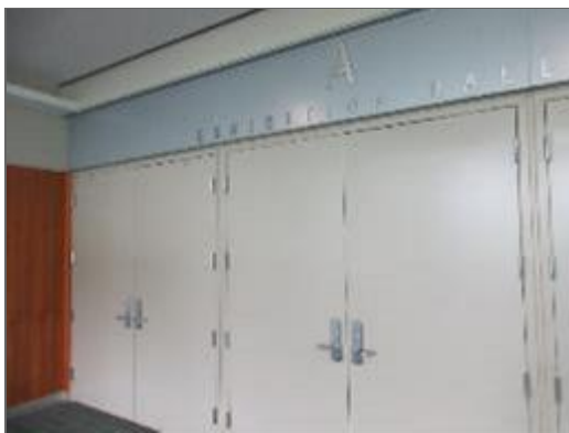
View of typical interior metal doors within the Site Building.
