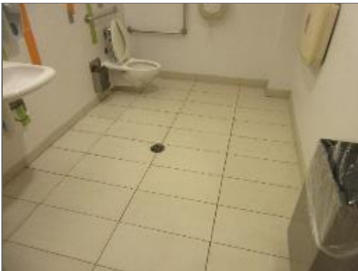
View of typical ceramic tile flooring in the washrooms.
