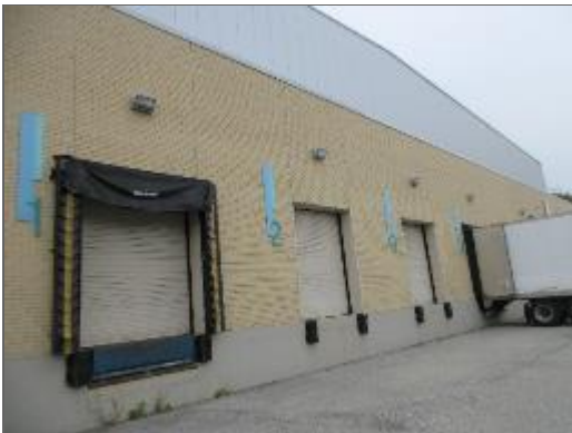
General view of the metal overhead rollup doors noted on the west elevation of Site Building.
