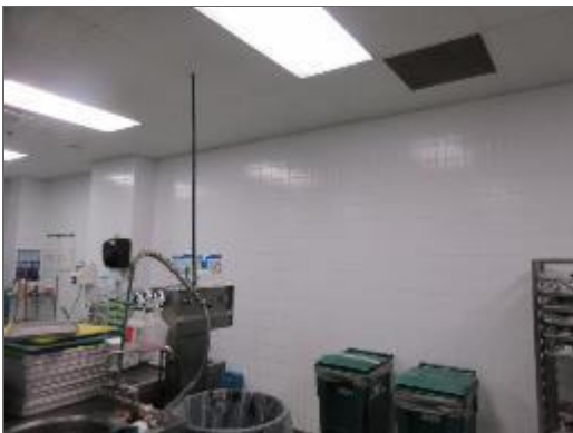
General view of the ceramic tile wall finishes within the kitchen.
