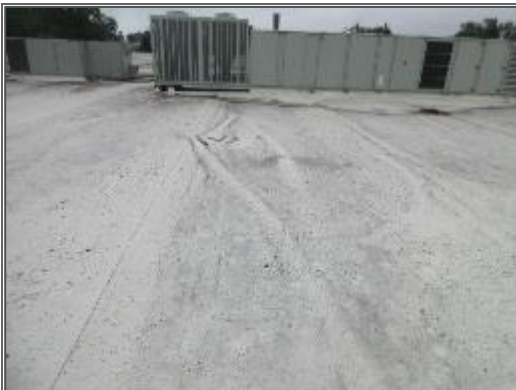
View of wrinkling in the TPO membrane.
