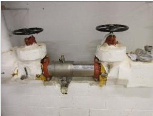
View of the backflow prevention device installed onto the main water line.
