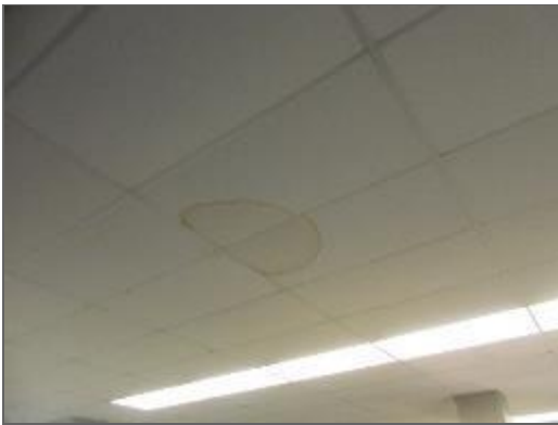
View of moisture-stained ceiling tiles in the office area of the Site Building.
