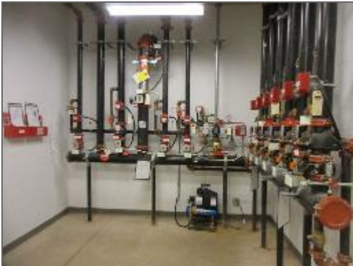
View of the fire sprinkler risers and shut off valves serving the Site Building.
