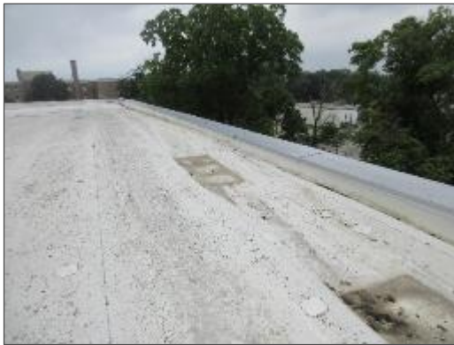
View of metal cap flashings at the roof parapet of the Site Building.
