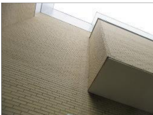
Close-up view of the brick veneer masonry on the south elevation of Site Building.
