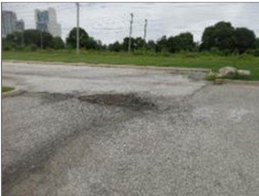
Typical view of deterioration and a pothole at the west asphalt-paved parking area.
