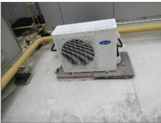
View of a typical air-cooled split condensing unit serving the Site Building.
