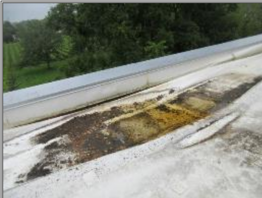
View of wrinkling and water ponding on the TPO membrane.
