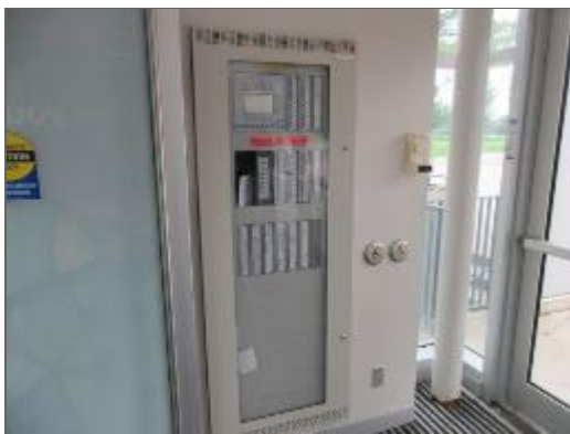
General view of the fire alarm annunciator panel at the main entrance.
