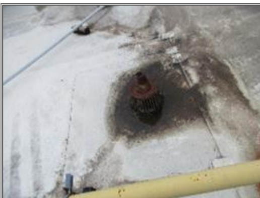
Typical view of a roof drain.
