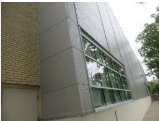
View of the metal wall panels noted on the east elevation of Site Building.
